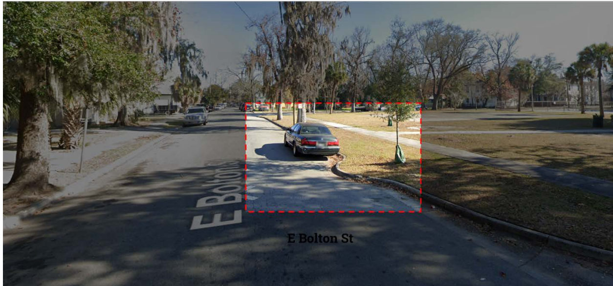
Image. The bell-shaped curb cut at the beginning of the curve to restrict parking on the driveway curve. Photo from Google, 2022.
