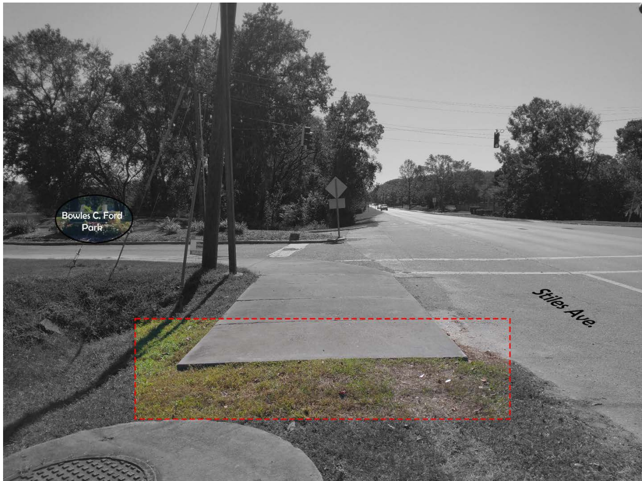
Image. Stiles Avenue as it intersects with Cloverdale Drive. Pedestrians have no protection when crossing the overly wide intersection, with no warning signs, walk signs, or painted walkways. The sidewalks aren't continuous either. Photo taken by EC, 2022.
