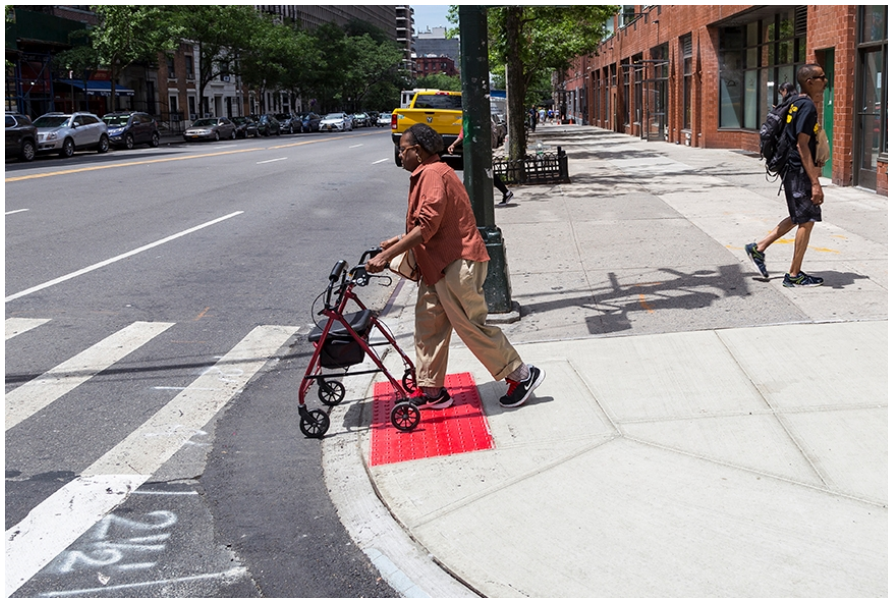
Image: Pedestrian Ramp at 96 th St, Manhattan, New York, NYC DOT Street Design Manual . Retrieved by EC, 2023.
