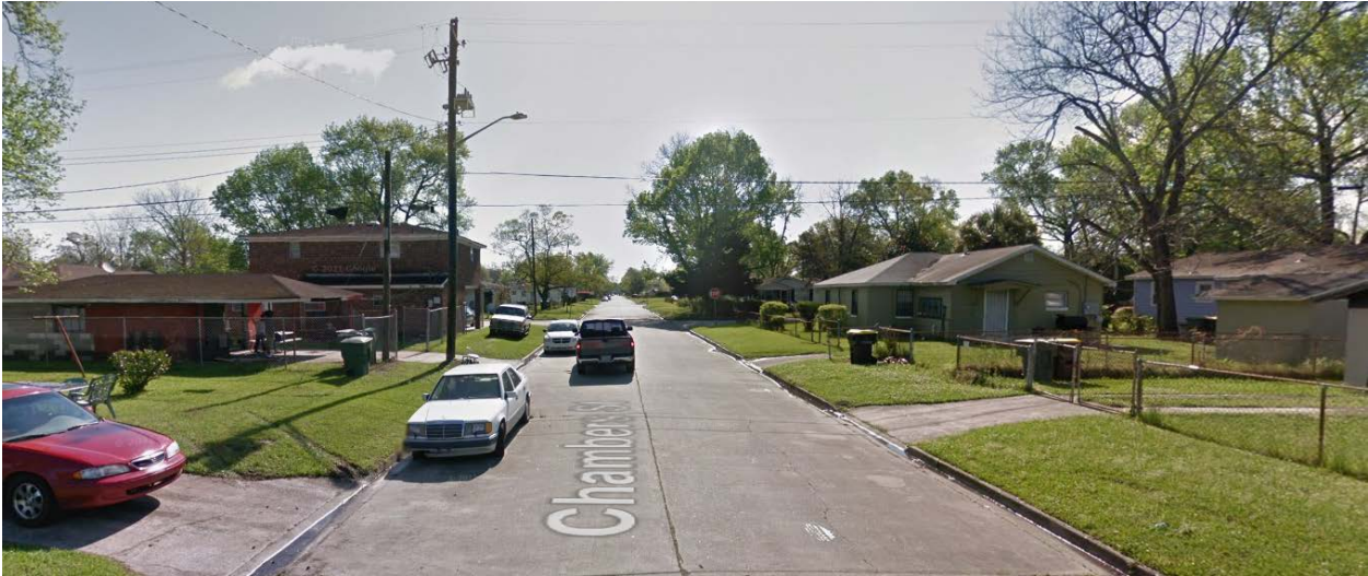
Image. Existing conditions on Chambers Street facing east towards Wexler Street. Photo taken by Google, 2022.
