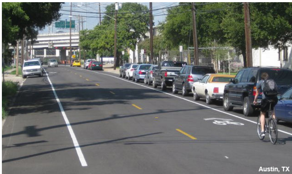
Source: NACTO Urban Street Design Guide (Image of Shared Lane Marking - Austin, Texas)
