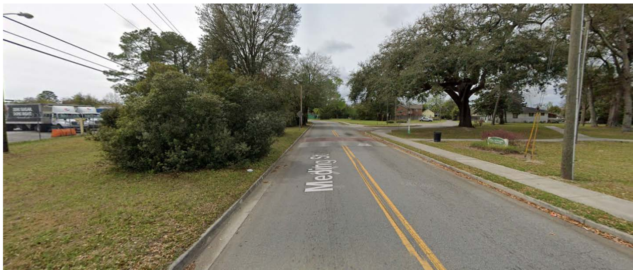
Image: Existing conditions on Meding St facing west. Photo taken by Google, 2022.
