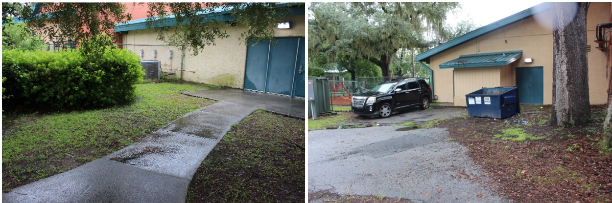
Images. Some pockets and corners within the complex are not very well surveillances as seen. Photos taken by EC, 2022.
