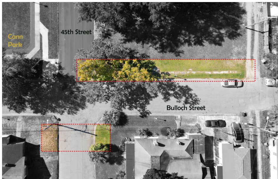
Image. Bulloch Street to the east of Cann Park, deteriorating sidewalk. Photo taken by EC, 2022
