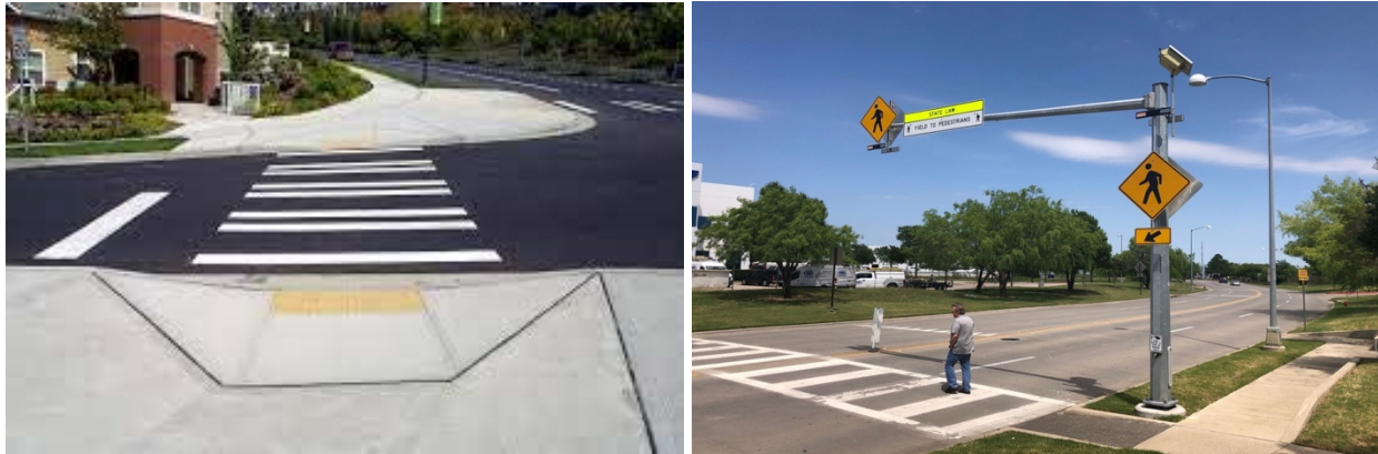
Images. An ADA-compliant pedestrian crossing (left) should be installed at residential intersections near Kennedy Park, and a push-button pedestrian crossing (right) could be installed at locations along West Gwinnett Street. Photos taken by Federal Highway Administration (left) and SmartCitiesWorld (right).
