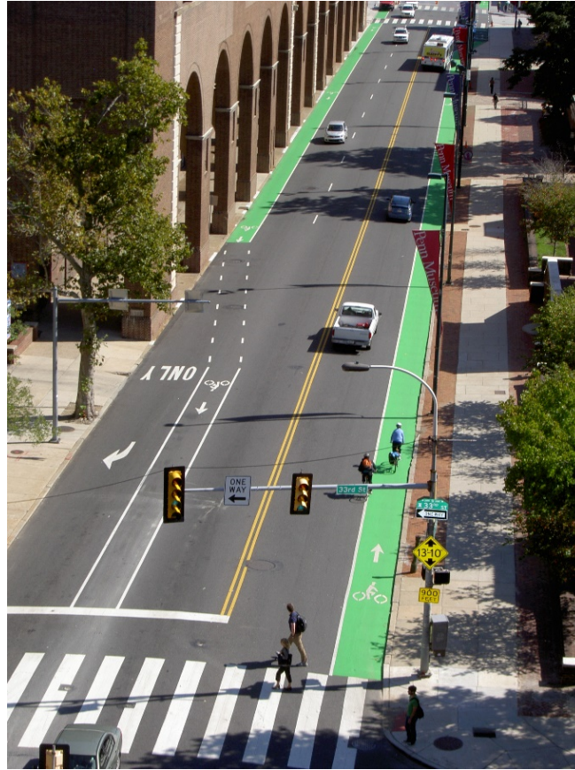
Image: NACTO: Urban Bikeway Design Guide (Image from Philadelphia: Durable Liquid Pavement Markings). Retrieved by EC, 2023.
