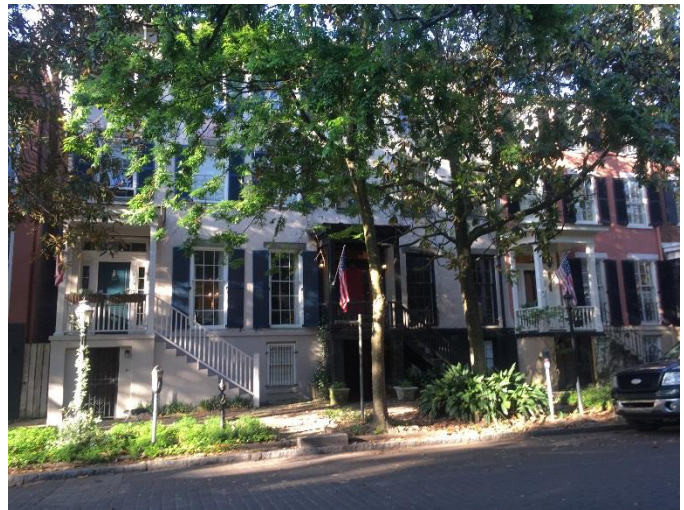
Jones Street has 47 DUA on this block
